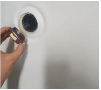
The backup heater connection is located on the flange at the bottom of the tank behind below plastic cover:
